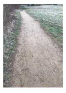
Either side are photos of the path. The path has a camber allowing water to run off. You can also see the colour of the material.
