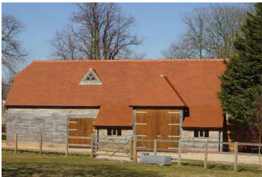
Recently constructed timber frame barn at Stargroves, East End
