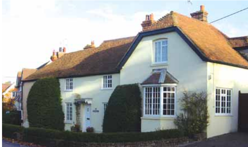
The Old Sun Inn, East End (early C19). Variable roof geometry, hipped, half-hipped dormer windows. Low height to eaves and ridge. Slate roof to rear. Painted render walls. Canopy on brackets over door. Windows in reveals
