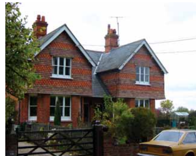
New Villa, Gore End. Slate roof, substantial chimney stacks. Decorative and plain hanging tile in bands
