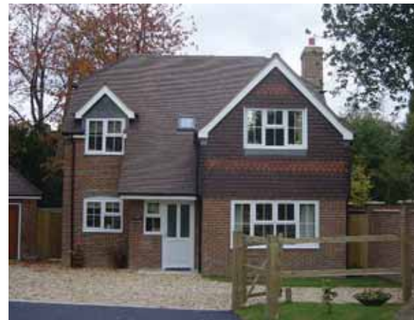
Acorn Cottage, Ball Hill. Small plot ratio, but well disguised by good landscaping. Variable geometry, half hipped roof, dormer window. Black rainwater goods, white facia. Well-matched bricks, band of blue brick at first floor level, rough arch plain and decorative hanging tiles. Small window panes. Garage set back behind building line.
