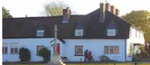
The Forge (C17) and The Court (C19), East End. Variable roof geometry, dormer windows, Chimneys. Low heights to eaves and ridge. Slate roof to rear. Painted render walls. Canopy on brackets over doors, porch over door. Triangle junction in foreground
