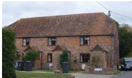
Beavers Lodge, Heath End (early C19, rebuilt as a terrace in 1998). Structure abuts roadway. Hollington brick and tile. Half-hipped roof, modern soldier lintels, modern porches reflecting traditional style
