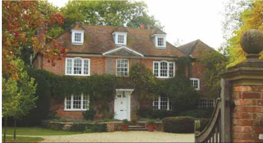
Vinnicks, Hollington (early C18) - formerly Hollington Farmhouse. One of the few three-storey buildings easily visible from the public highway. Garden walls and gates. Third floor built into roof void using dormer windows, so no overall increase in height of building. Substantial chimneys. Black rainwater goods. White window frames with small panes. Canopy over front door.
