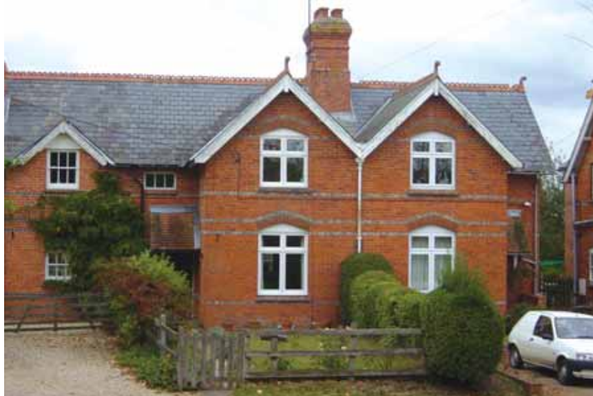
Rectory Cottages, East Woodhay. Good example of recent extension (left) using carefully matched materials and features. Ornamental ridge tiles. Chimney. Canopy over door. Fence and gates
