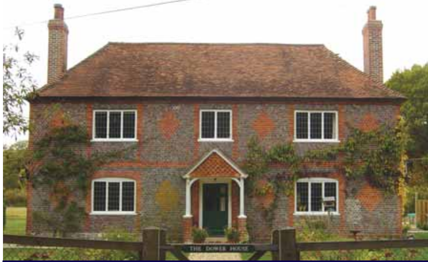
Dower House, North End. Hollington brick in header bond with architectural features in stretcher bond. Hipped roof in Hollington tile, chimney stacks. Windows in reveals. Porch with decorative hung tile.
